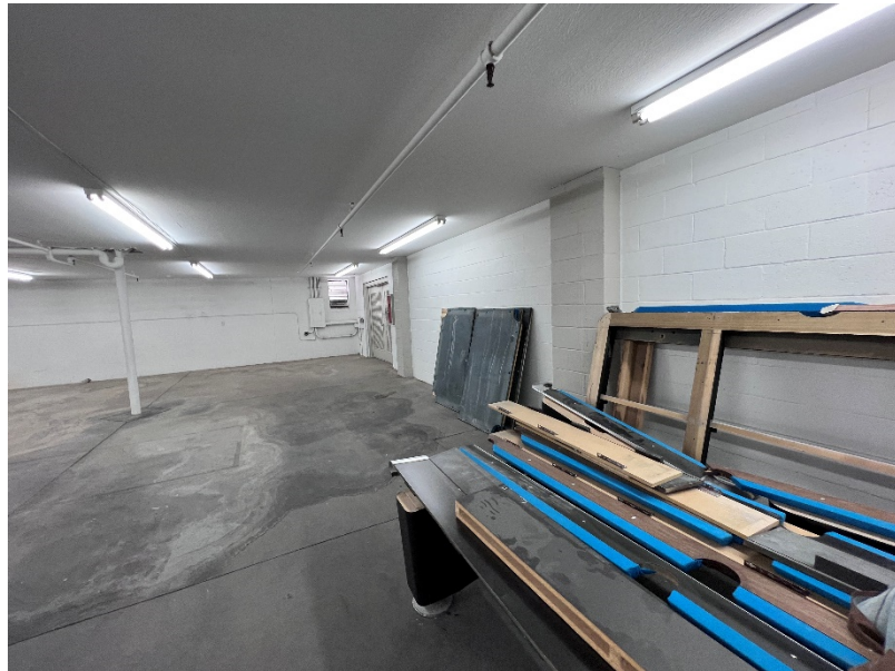
EXISTING PANEL 'C' TO BE DEMO'D AND REPLACED WITH NEW
